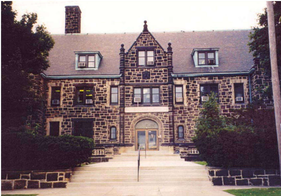
The former headquarters of the Harshaw Chemical Company headquarters is now part of the Cleveland Clinic on East 97 th Street, Cleveland, Ohio. The black stone construction is a unique architectural feature in this neighborhood in Cleveland. Photograph used courtesy of "The Nuclear Traveler." [1]
